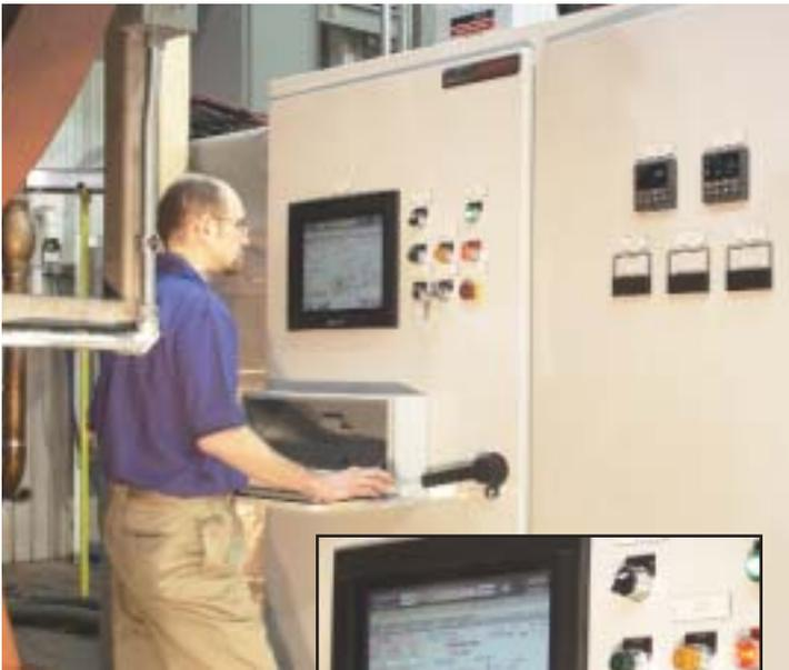
Technicians control and monitor Ipsen's heat-treating furnaces using a computer and display from CTC, a division of Parker-Hannifin Automation. The computer and display are flexible enough that Ipsen could make the current controls look like their older ones, but with more capabilities.
